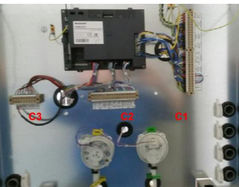
Each boiler has 3 terminal strips (C1..C3) and 5 cable guides.
